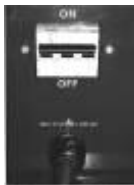
32 A D curve circuit breaker
